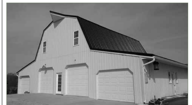
Wayne and Pamela Fry, built some new additions and remodeled their shed at West State Highway ZZ in McFall.
