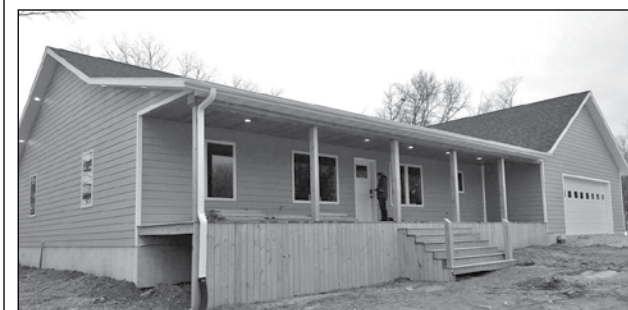
Koltyn and Mychelle Smith constructed this new home with a large deck on Monson Street in Bethany.
