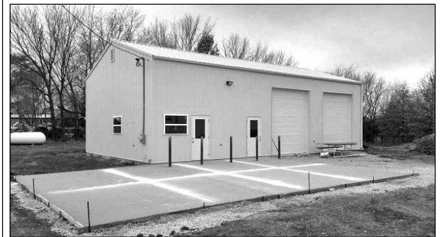
Max Daniel and Megan Wise built a new Laundromat with a 37 x 24 parking lot off Highway N in Blythedale.
