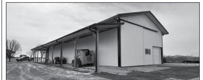
Jerad and Victoria Vandiver moved, upgraded and expanded on an old shed on West State Highway P, McFall.
