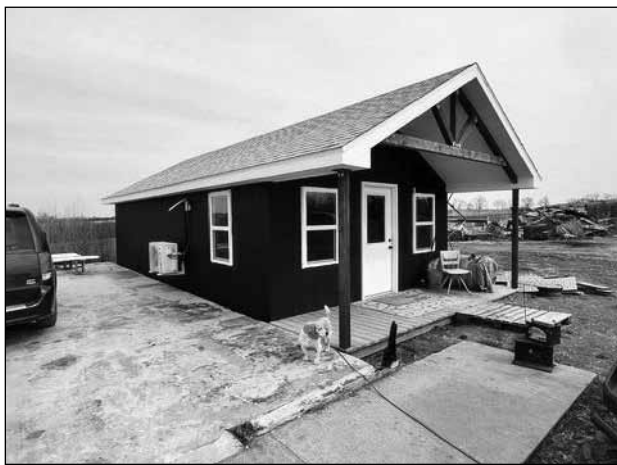
Rusty and Sarah Clark constructed a new tiny house and cattle shed on West 125th Avenue in New Hampton.
